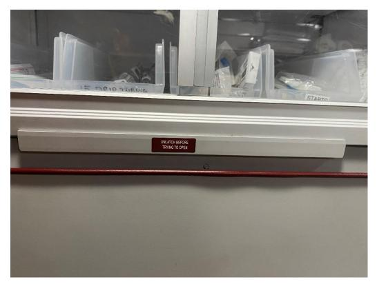
1.1) Exterior locking mechanism for patient compartment cabinet to match below
